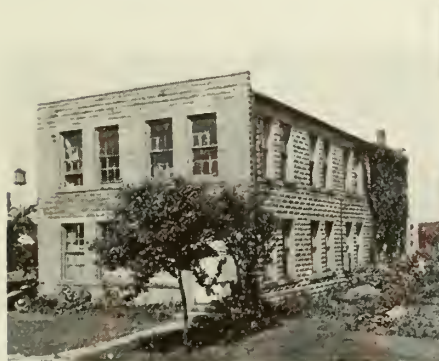
Libertyville Textiles, Inc. North Fifth Street
